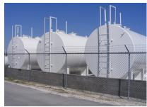
Series 740 UVX was chosen to protect the exterior of the Albert Ellis Airport Fuel Storage Tanks in Fountain, NC because of its abrasion resistance and exterior weathering properties.
