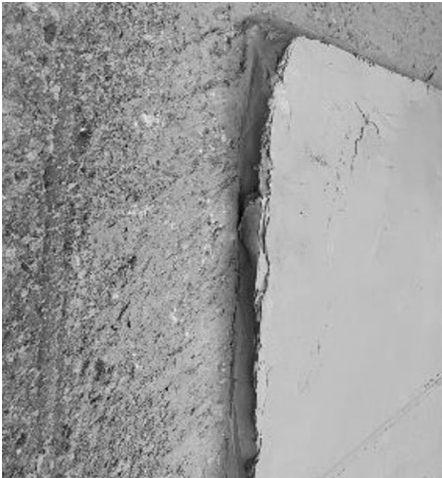
Final edge condition is depicted in the photo above.
