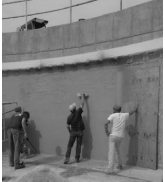
The use of 3/8" plywood is used in the photo above
