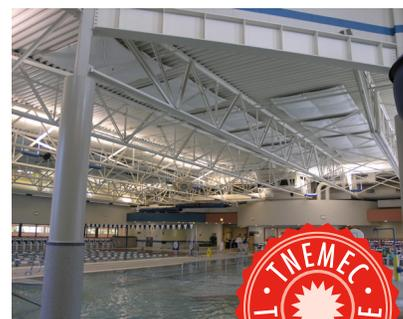
Various Tnemec coatings were used to protect the concrete block walls, reinforced concrete floors, structural steel framing, galvanized roof decking and steel joist roof framing at the Oakbrook Family Aquatic Center in Illinois.
