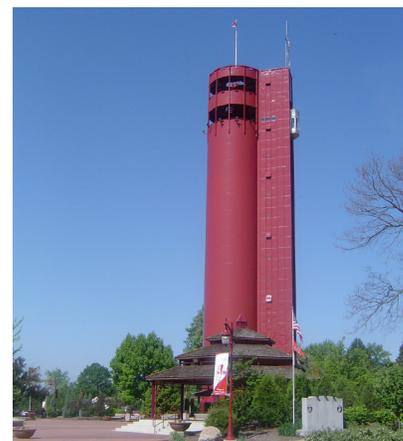
Series 700 HydroFlon, a fluoropolymer polyurethane finish with excellent color and gloss retention, protects the exterior of the standpipe in Peoria Heights, IL.
