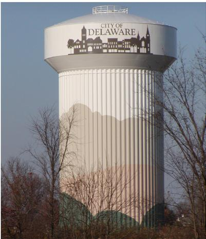
Series 700 HydroFlon, a fluoropolymer polyurethane finish, protects the exterior of the Southeast Highland Elevated Tank in Delaware, Ohio.
