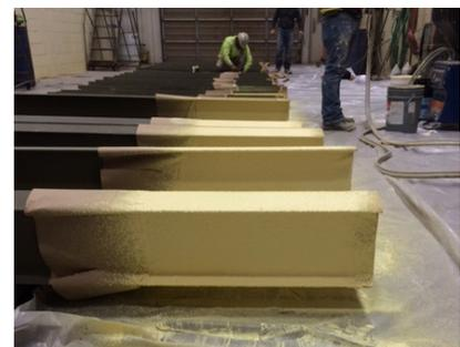
Tnemec’s thermal insulating coating, Aerolon, was applied to steel beams for a Pennsylvania student union to mitigate thermal bridging and limit condensation within the building.
