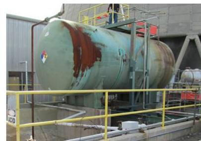
The location and elevated temperature of this sulfuric acid tank caused accelerated corrosion on the steel before being repaired and recoated using Tnemec's innovative thermal insulating coating system, Aerolon.
